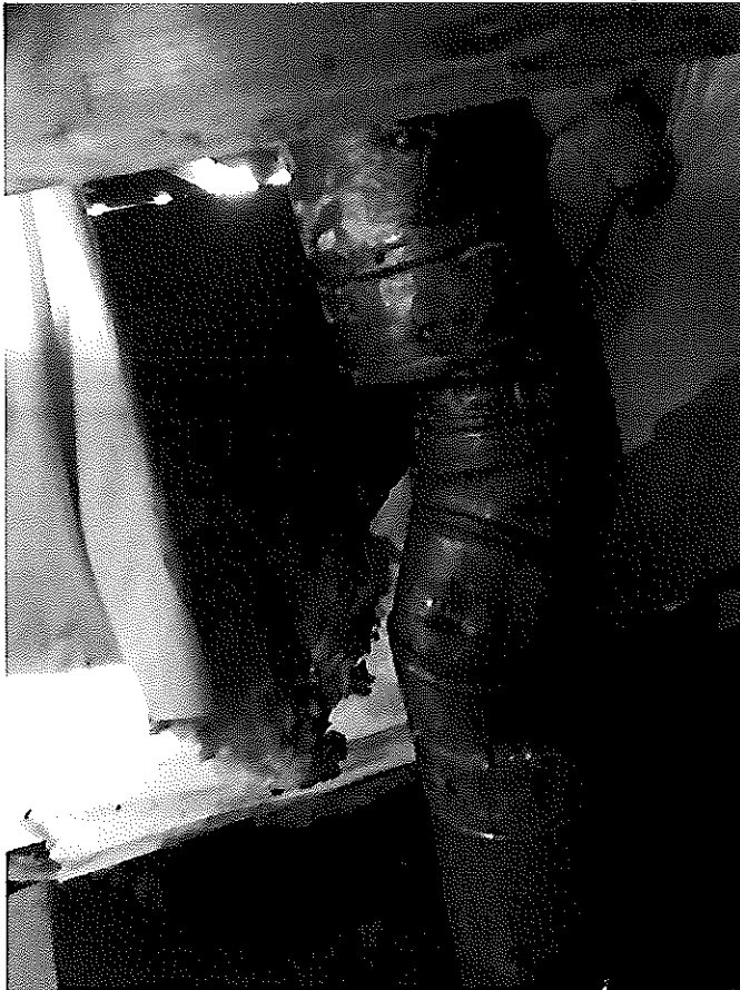
Pipe above water heater – Bill fixed pipe put still has leak in roof
